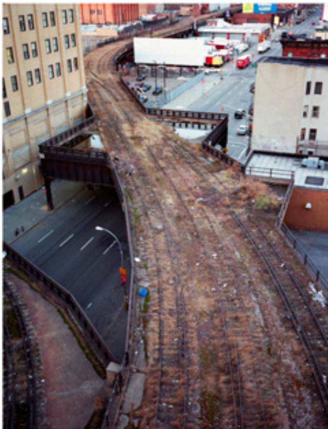
High Line – Before
