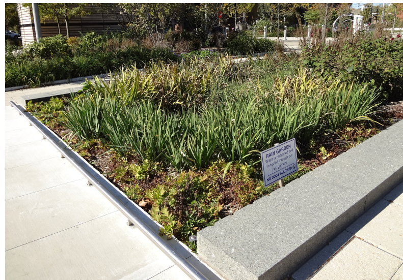
Figure 4 Example of rain garden, image by ETM
